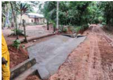
Rainwater channelling and construction of residential entrances ©APDS
